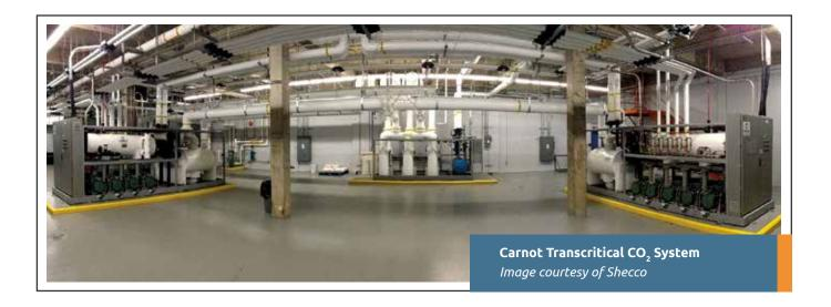
eight heat recovery units, two gas coolers, and about 2,474 kg of CO<sub>2</sub>. 113 Other benefits of the system include 60 percent less space needed for refrigeration equipment, 10 percent reduction in maintenance costs compared to a conventional system, and no cooling tower required. 114 The system recently won an Energia Award in the Existing Building – Institutional Sector category from the Quebec Association of Energy Efficiency. 115
